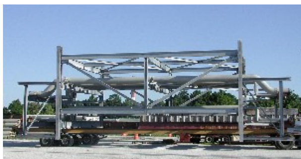
Figure 6-1 Example of a 9m wide x 18m long pipe rack module being transported to site.
