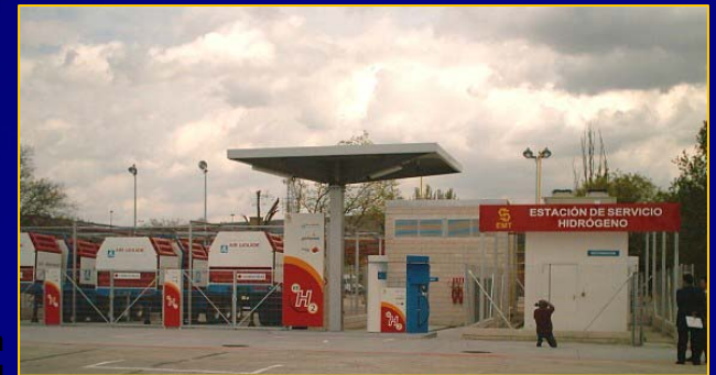
NG reformer station Madrid
