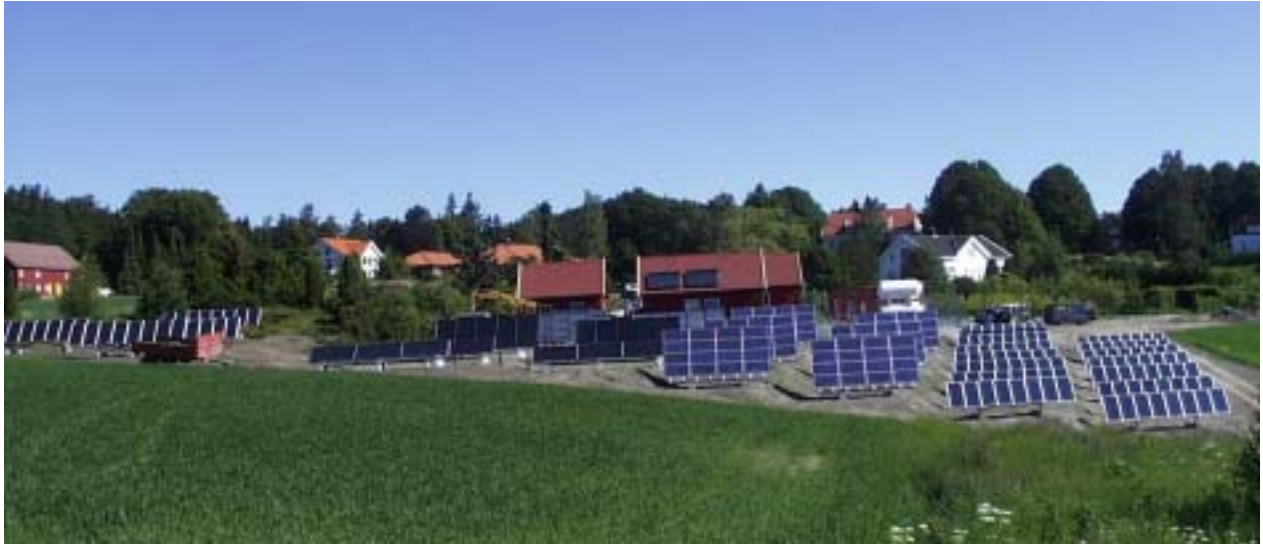
Figure 1: An overview over the Energy Park at Dømmesmoen, Grimstad
