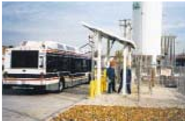
Figure 5: CTA hydrogen fueling facility in Chicago
