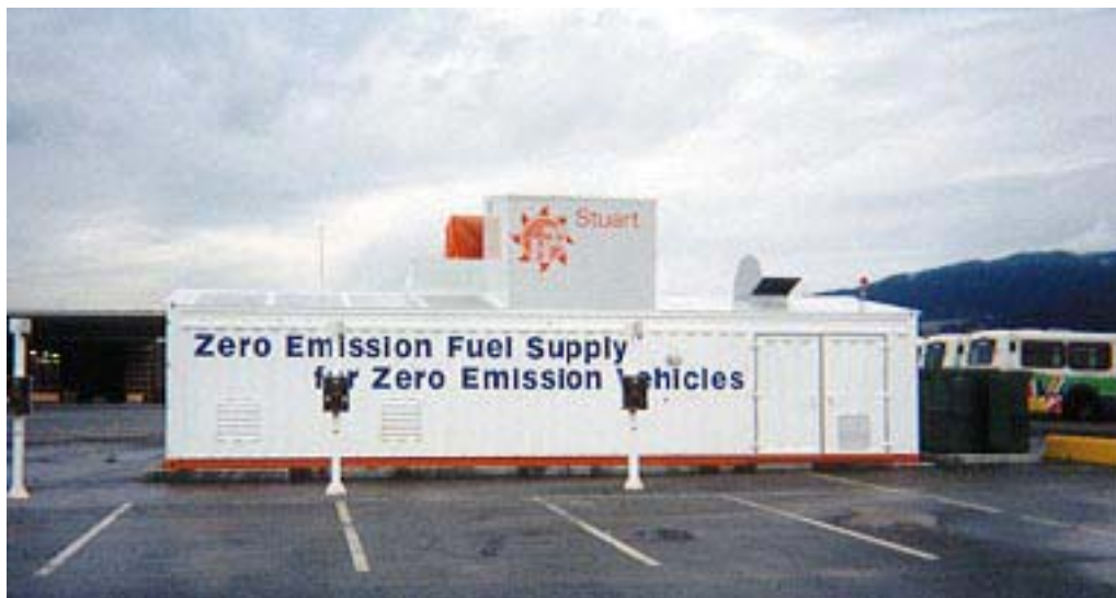
Figure 7: Hydrogen refueling station at Port Coquitlam
